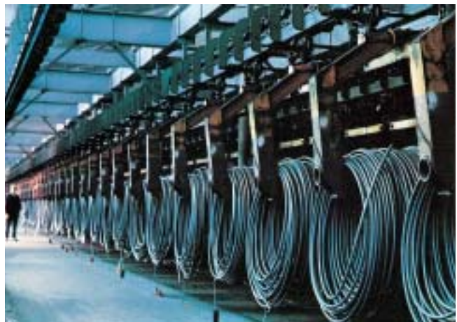
Power & free conveyor system
