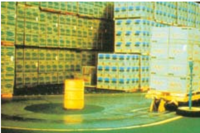
Towline conveyor system for stocking
